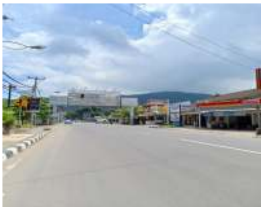
Figure 2 Condition of Senggigi Areas Post Lombok Earthquake
